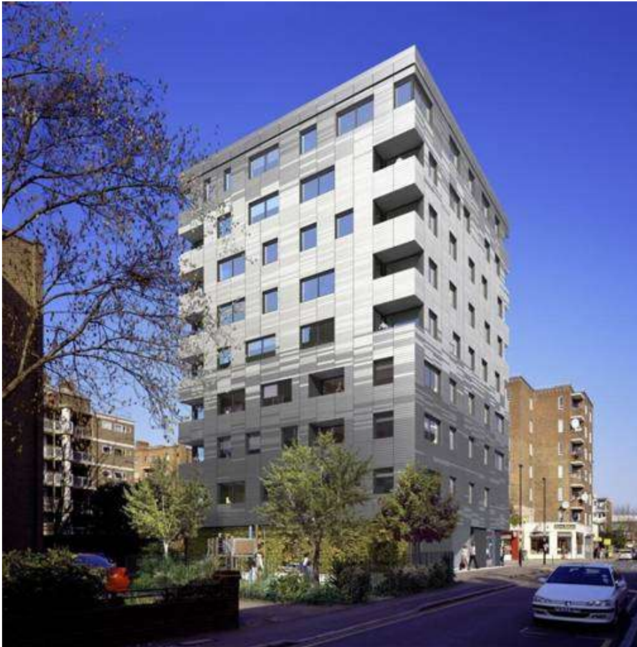
Murray Grove Building, London, 9-storey
